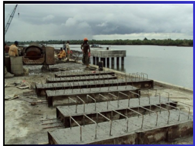
Precast beam for reinforced concrete apron behind shore wall
