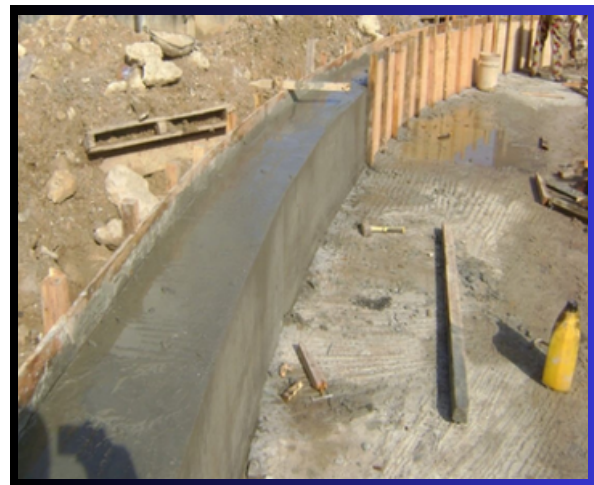
Complete reinforced concrete apron behind shore wall
