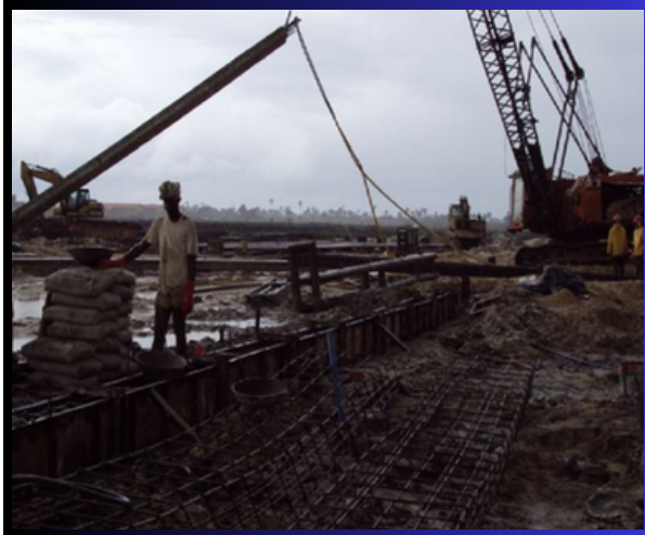
Crane lifting 14m of sheet pile to be installed
