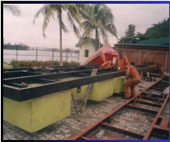
Construction of floating jetty for American Embassy
