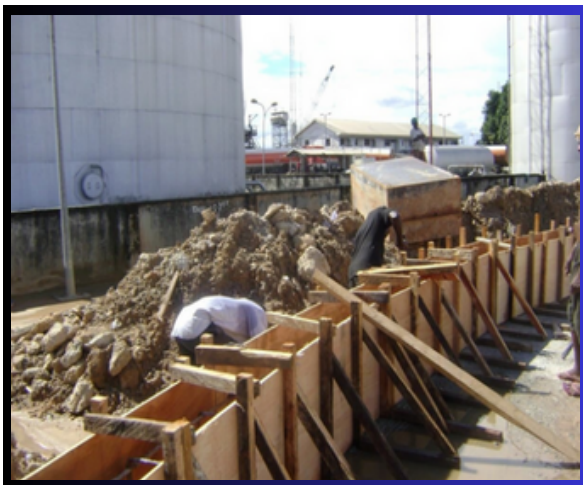
Formwork for ring beam construction at Port Harcourt Conoil Depot
