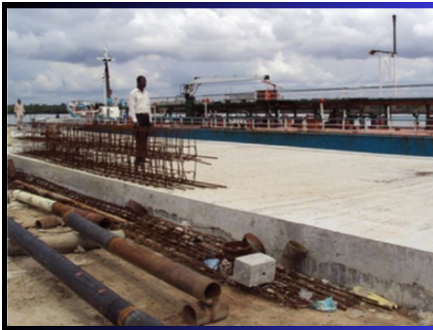
Complete reinforced concrete apron behind shore wall
