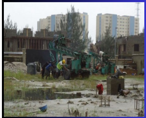
Construction of Pile Foundation (Bore Pile) at Banana Island, Lagos
